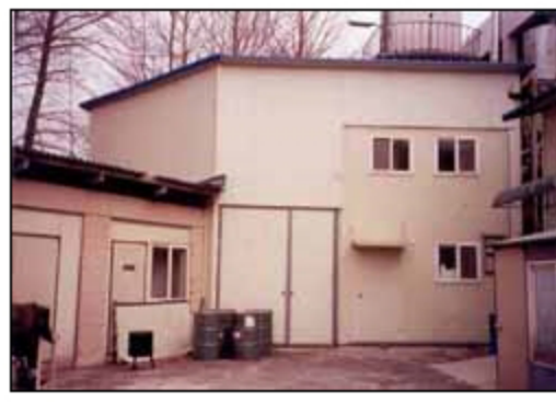
Fuel Additive Laboratory for Heavy Oil(Top)
